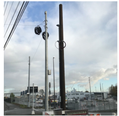
Newly installed signal pole for Duwamish Longhouse
