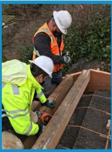
SDOT staff rebuilt the stairway at 10th Ave S & S Donovan St in Q2. To keep our stairways safe and accessible, SDOT inspects the condition of each public stairway across the city and identifies repairs. Repairs range from replacing the handrails to replacing the stairway altogether.
