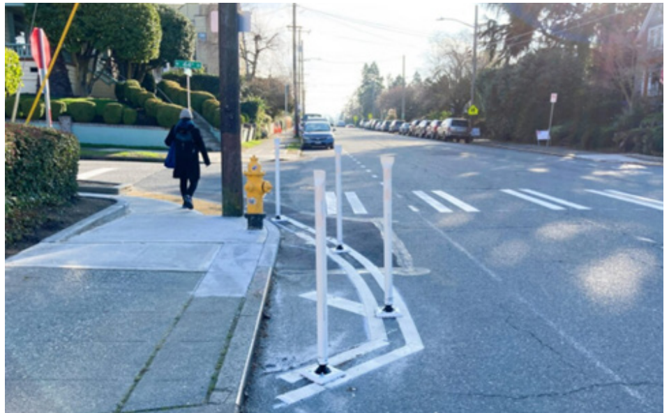
Most of the new marked crosswalks will include "paint and post" curb bulbs like the photo above on the west side of 3rd to make the distance to cross the street shorter and make people walking more visible to people driving.
